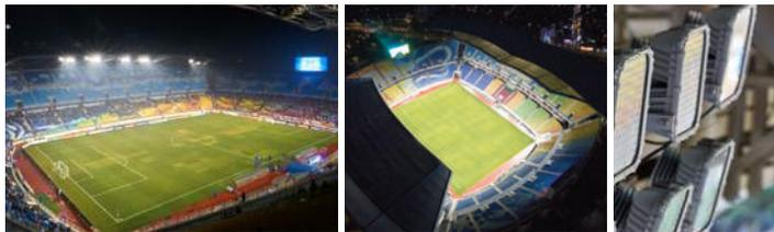
The Suwon World Cup Stadium which was fitted with 120 units of SUFA-A 1.2kW is a professional soccer stadium that was the first example of such an installation in Korea. As with other stadiums, the lighting was installed with the event lighting function available.
