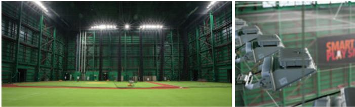
“S” baseball team has installed MAHA floodlights at its indoor practice stadium. This was a replacement project for products from global brand “M”. The plan is to provide wireless control capability and a maximum lux level of 1,200.
