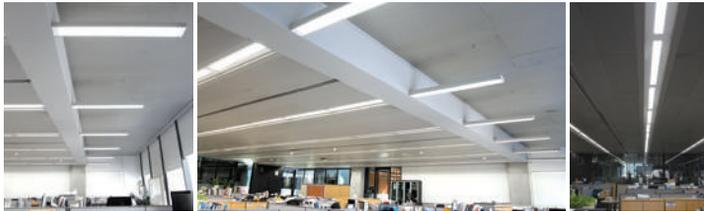
Obsolete office lights have been replaced with new LED's through an initial lighting trial and subsequent full swap on the 9th and 12th floors of an 8 years old building. Work environment, eco-friendly corporate image and energy usage levels have been optimized or enhanced.
