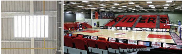
England's Leicester Riders Stadium has installed IBL high bays to light up its interior. Through the indirect reflection of light onto the court and into the eyes of players and audiences, the IBL avoids any direct beams from glaring into any eyes.
