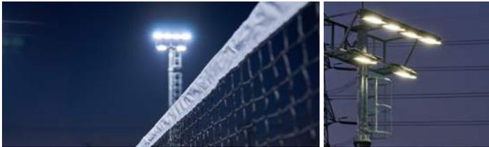
The MAHA products installed at Ulju Cheongyang Dongcheon have been installed in a high-mast two-tier structure and thanks to lighting cut-offs possible by MAHA products and their overall uniform light output, we have been able to achieve an excellent level of uniformity at the tennis court.
