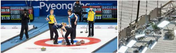
This project was an installation case where a total of 92 units of SUFA-A 1.2kW were installed that have a color temperature of 5700K. Also, a 90Ra high color rendering product was introduced, and the SUFA-A product was installed along with a remote driver separate from the power supply device, which was installed on the product.
