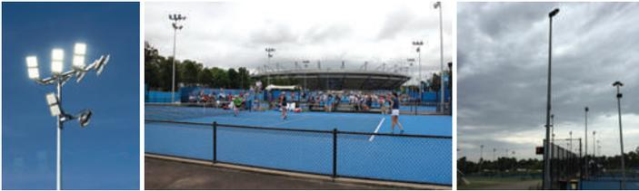
In June 2014 Lamptech approached the Sydney Olympic Park Tennis Center to discuss replacing the existing metal halide lighting system with GigaTera LED's. This project marked the first installation for a broadcast quality sporting facility in Australia. The project consisted of a total of 120 Sufa 400W fittings installed at 6 courts with the primary goal of increasing existing light levels while achieving power savings and the secondary goal of lowered maintenance costs.
