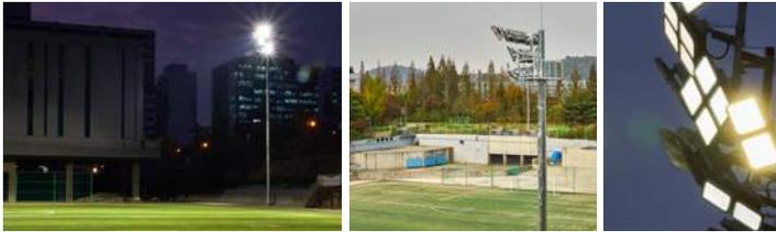
On each of the posts of the lighting towers that are 18M tall, we installed 6 units of the SUFA 800W product and 4 units of the SUFA 400W product. There were 4 lamp posts, which means that a total of 42 units SUFA sports lighting were installed.
